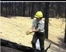
**Mulching** will stabilize the soil surface to prevent movement of soil particles and loss of seed. Use straw or grass hay mulch. Apply mulch at 70 lbs/1,000 sq. ft. (about 43 bales per acre). Use weed free material. Do not fertilize the first year. Use netting to keep the mulch in place on small areas of steep slopes. Hydro mulching and seeding is very expensive, but it can be accomplished in one operation.
