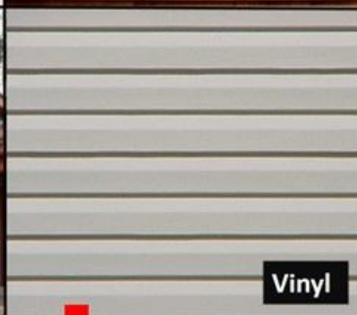
Melts at high temperatures
